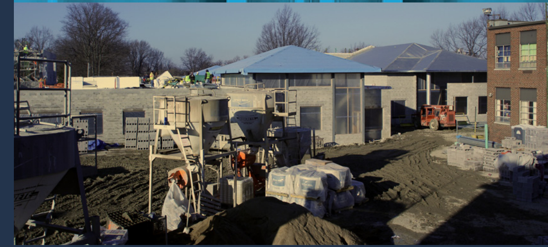
Construction at the Shoreview site, January 2012
